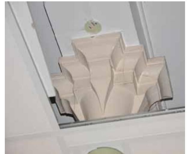
*Images from the basement. NB: New stud wall scribed around existing panels. All fireplaces retained. Capitals to columns retained behind replacement suspended ceiling.*
