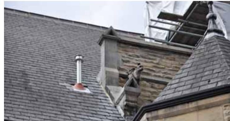
*Existing heaters and flue to the roof. Proposed to be removed and replaced with a ducted solution. Below: Existing (historic) flue extract.*
