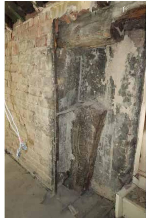
Images of First phase Cross Wing. (a,b) Including fireplaces, c) modified mullion windows to rear, d) Inserted wall, e) First floor chamber with fireplace and f) Remains of post structural elements. Overleaf, more images of timbers and stone flagged floor below 19th century concrete floor.
