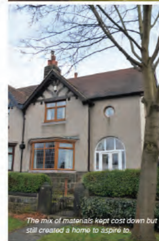
The exclusive development at Park Side used inspiration from the early Yeoman houses and reflected these in the proportions, materials and features such as mullion windows and finials to the roof.
