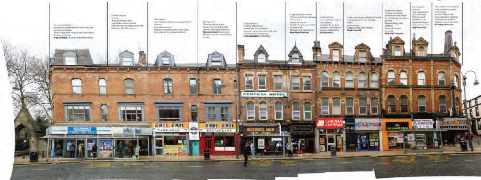
29-51 New Briggate. The extent of disrepair, inappropriate change, vacancy and loss of historic architectural detail is having a negative impact on the area and offers scope for significant enhancement through heritage-led regeneration guided through the proposed TH grant scheme
